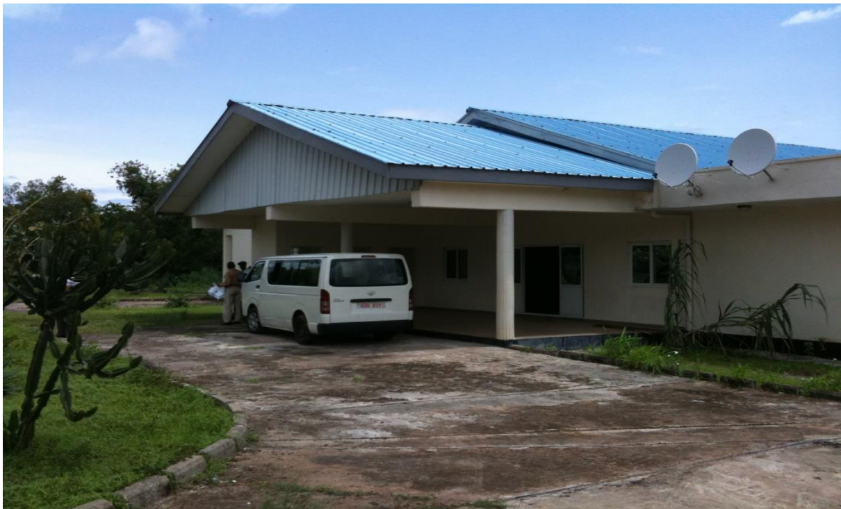
View of the Recreation centre and Reception with drive leading to the carport.
