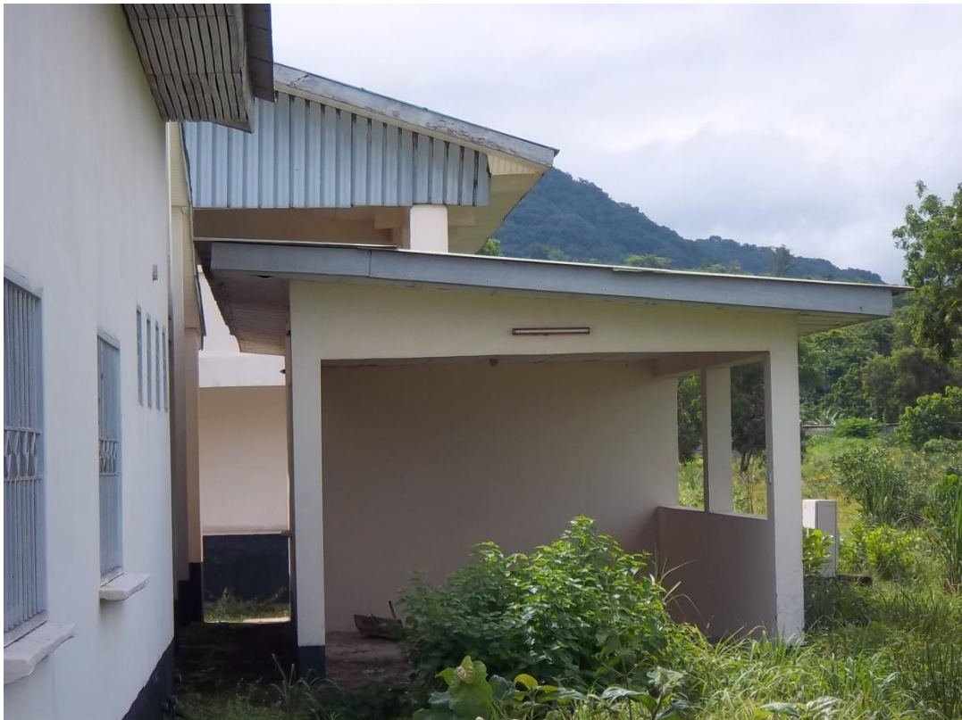
Front view of the Boat house near the Squash court building.
