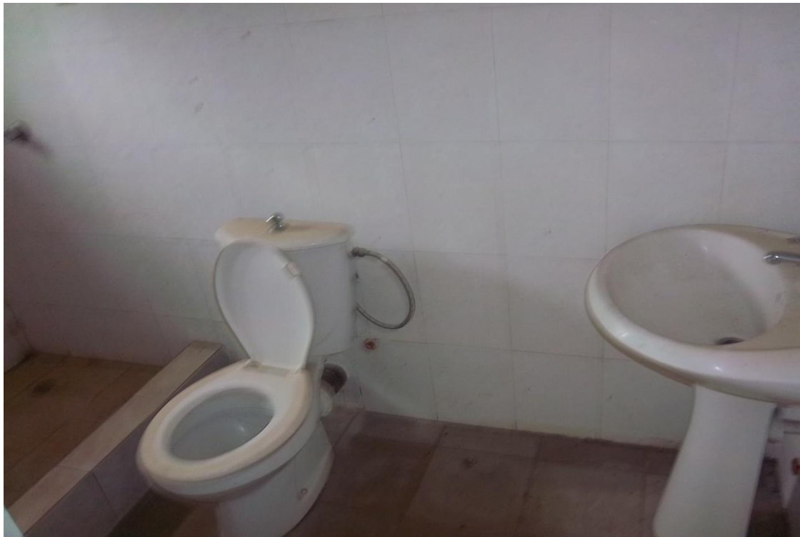
Internal view showing the shower, water closet and wash hand basin
