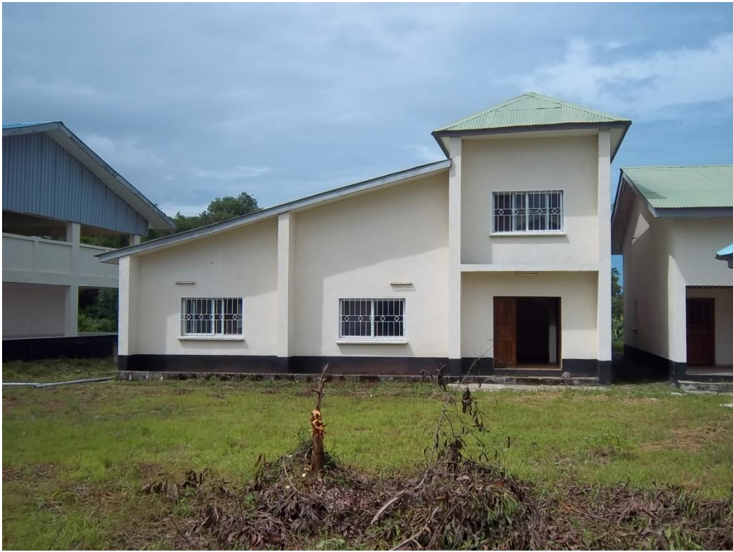
Front view of the Squash Court and Fitness Centre
