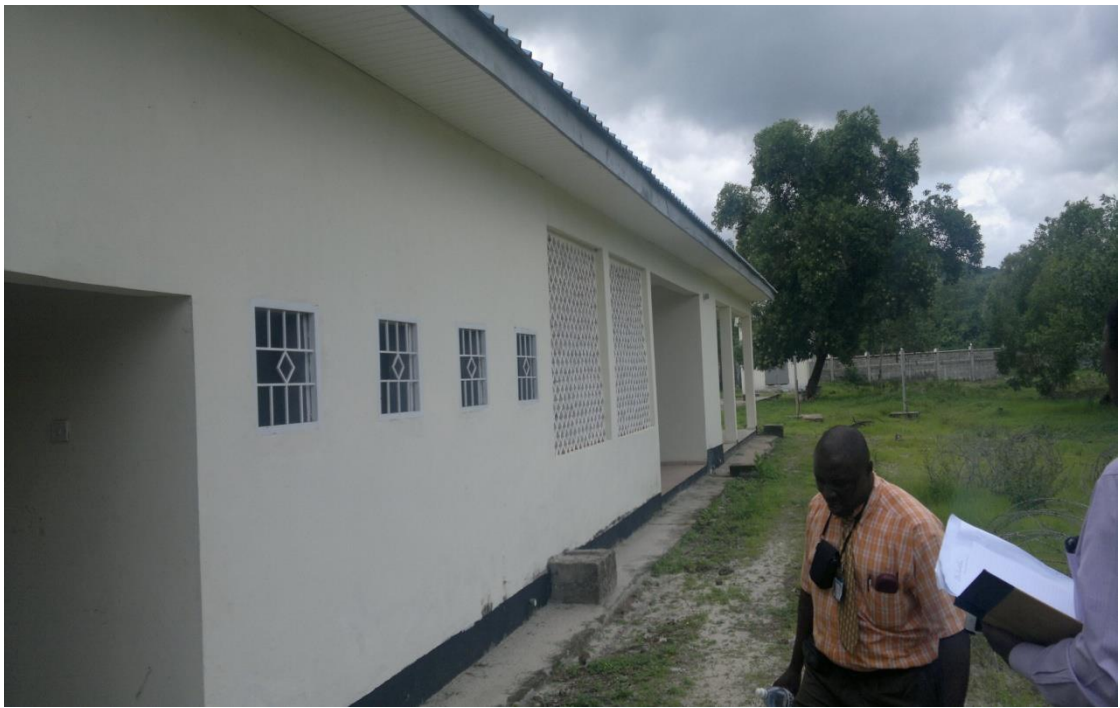
Left side view of the Recreation centre and Reception building
