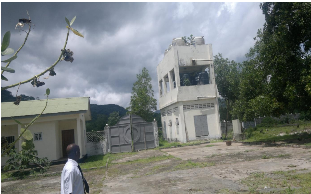
View of the generator house and pump room with the exit gate and part of the security post
