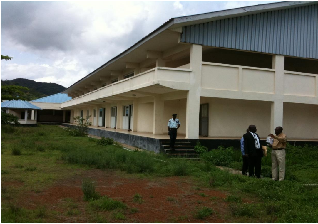
Left side view of the Conference/Training centre/Multi-Purpose Hall
