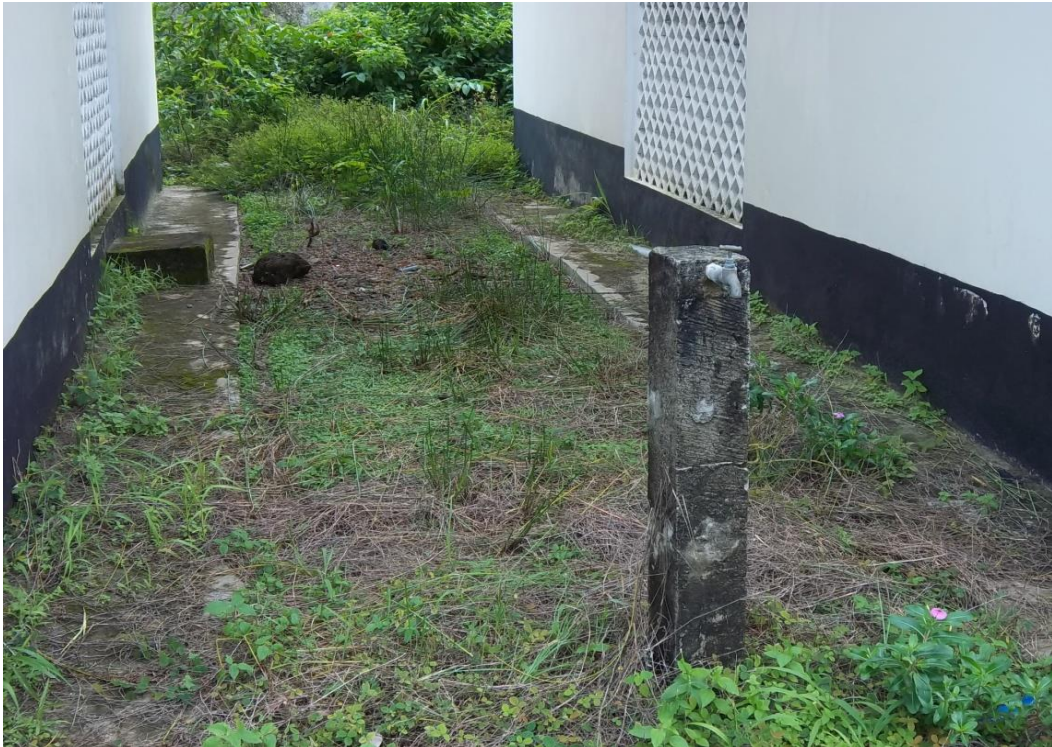
Stand-by tap supported on concrete post for watering the landscaping.
