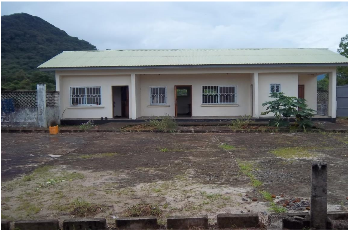
Views of the Security post
