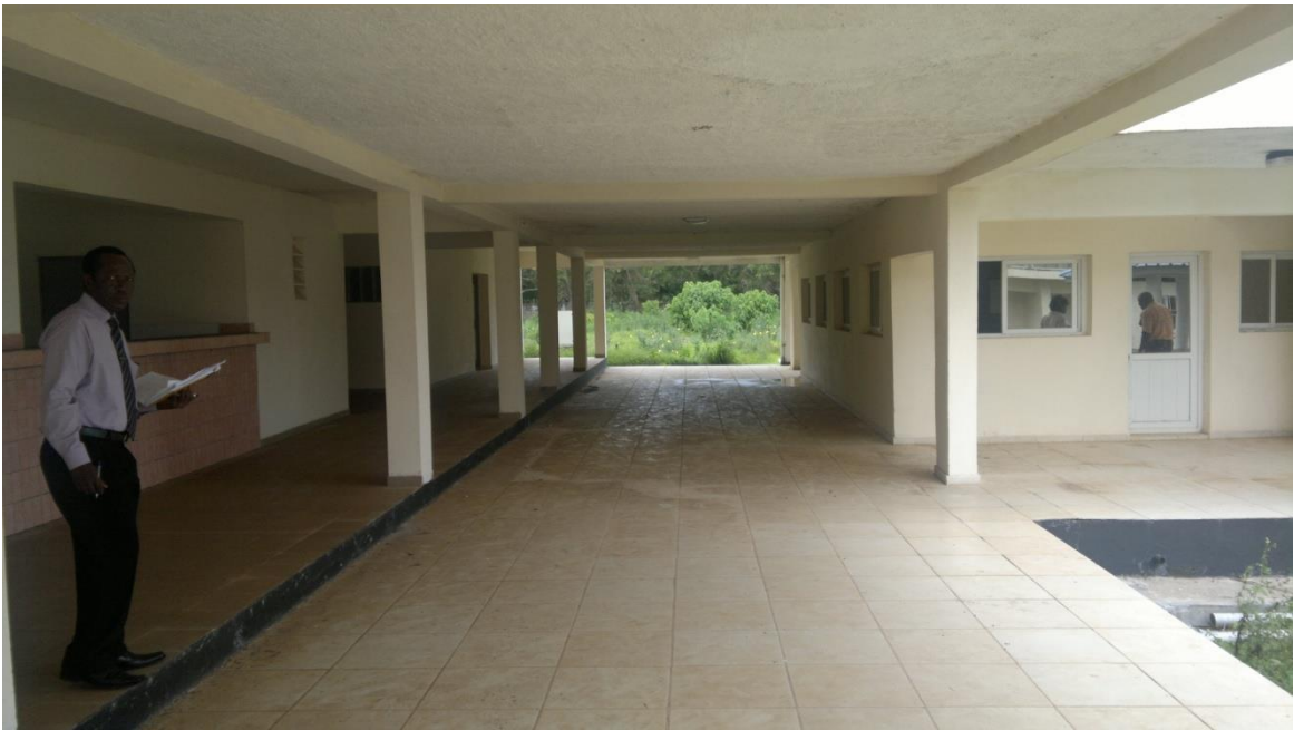
View showing the corridors in the Recreation centre and Reception building
