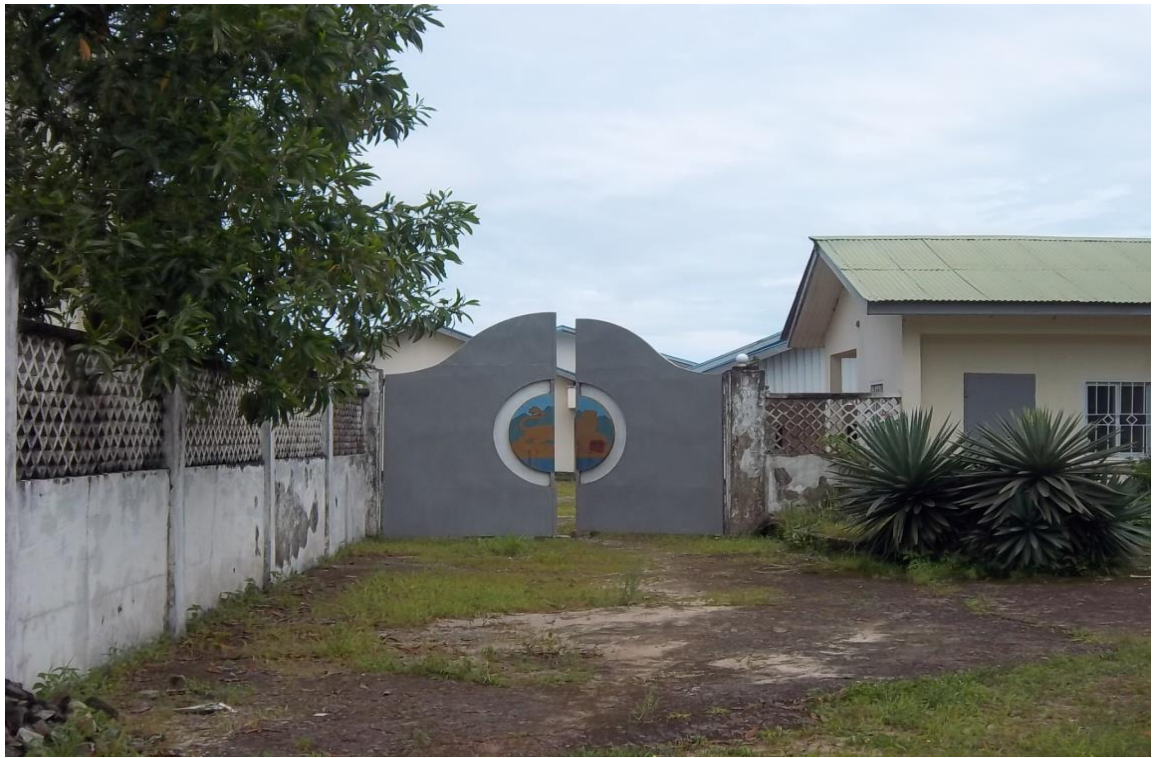
View of the Exit gate
