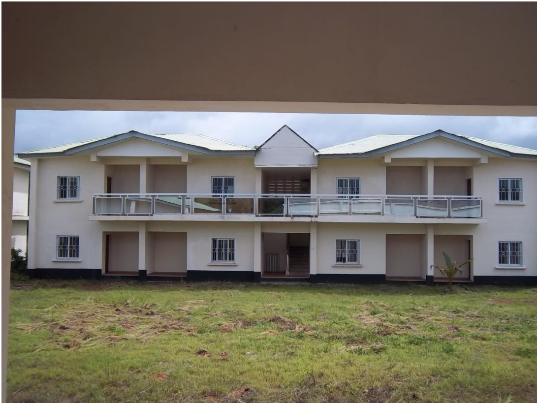
Front view of the one bedroom apartment block
