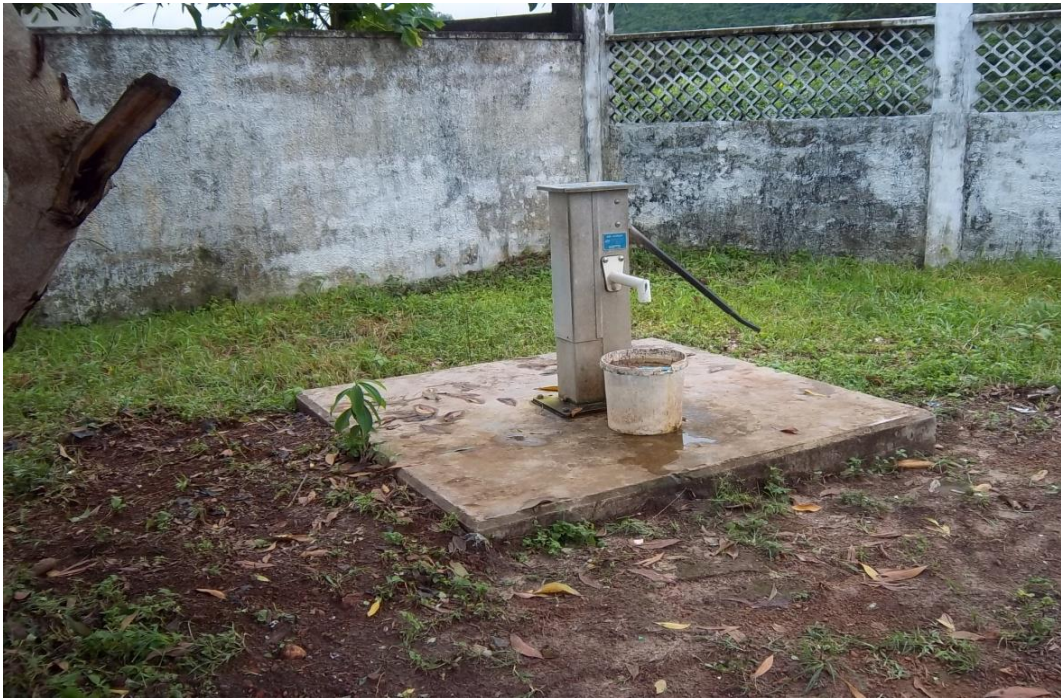
Water well constructed on the left end of the entrance gate.
