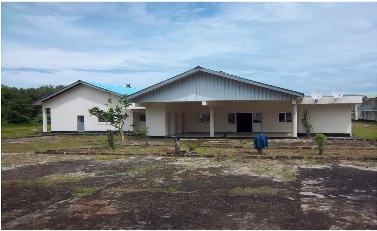
Front view of the Recreation centre and Reception building with the Medical unit at the far right
